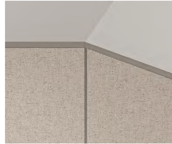
Detail of shaped panel for sloped ceiling
